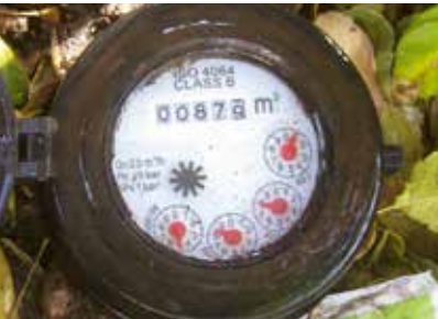
Example 2 - this is a ¾” meter measuring water for the groundskeeping. It reads 879.0885 m³.
